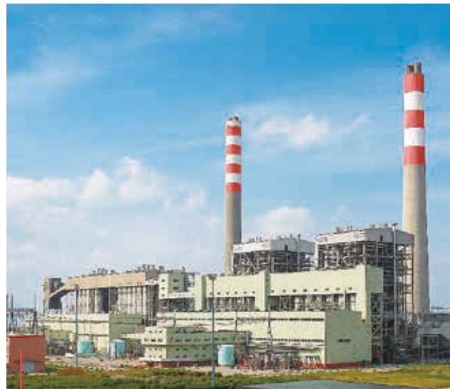
Jinwan Power Plant successfully reduces emissions after a major overhaul.
