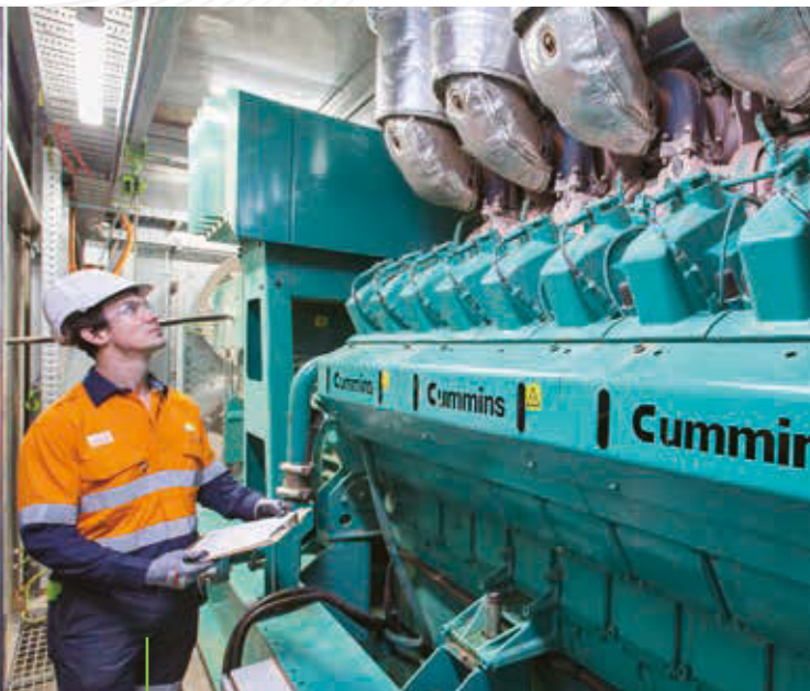
EDL expanded the Agnew Hybrid Renewable Microgrid with 18-MW wind and 13-MW battery infrastructure in 2020.
