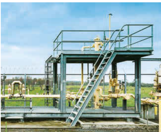
MG implements extensive network maintenance works to ensure reliability.
