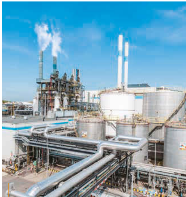
AVR's facility is helping to dispose of hospital waste materials during COVID-19.
