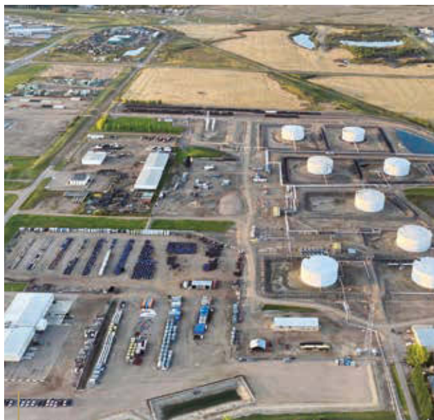
The oil processing facility at Lloydminster Terminal forms part of HMLP's expanding footprint in Canada.
