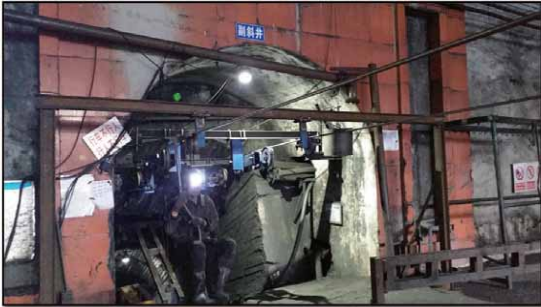
Figure 9-6: Auxiliary Decline of the Xiejiahegou Underground Coal Mine
