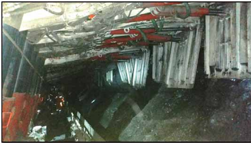
Figure 9-10: Longwall retreat mining at the Xiejiehegou Underground Coal Mine
